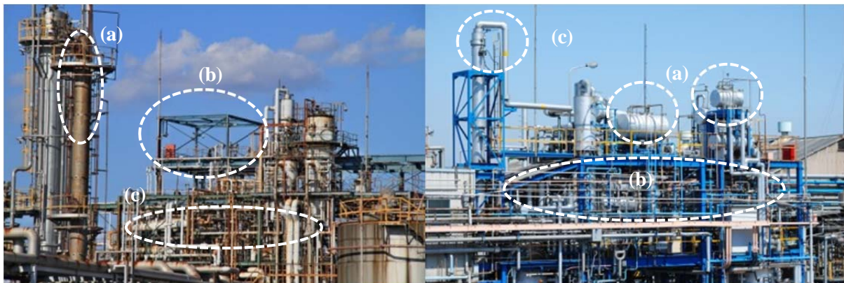
#1: (a) Tower, (b) Frame, (c) Pipeline
