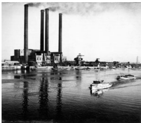
Fig. 1. The ghost chimneys in Japan, part of the Senju Thermal Power Station (1926–1964) maintained by the Tokyo Electric Power Company. [Used with permission from Adachi City.]
