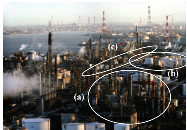
#1: (a) Processing Unit, (b) Tank Yard, (c) Pipelines
